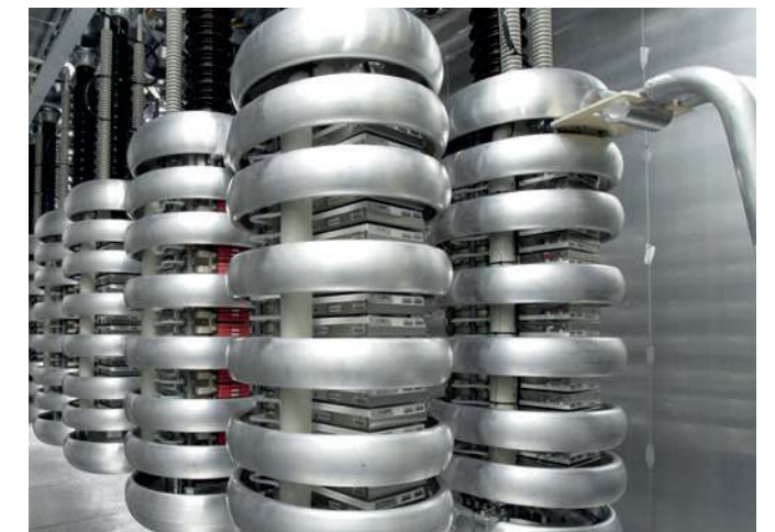
Fig. 5 Standard IGBT valve for VSC, HVDC and STATCOM
