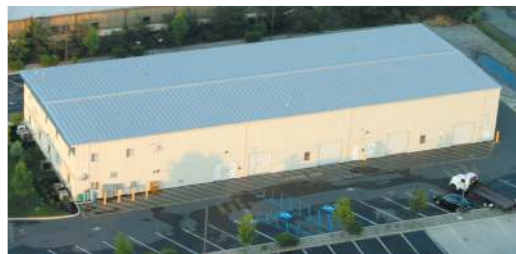
Farmingdale, NJ facility
