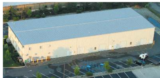
Farmingdale, NJ facility
